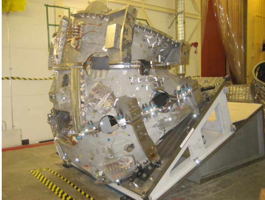
Figure 2. NCSX Modular Coil Half-Period Module under assembly
